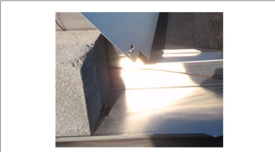
Fig. 2.1.1.11b. Flanged pedestal
