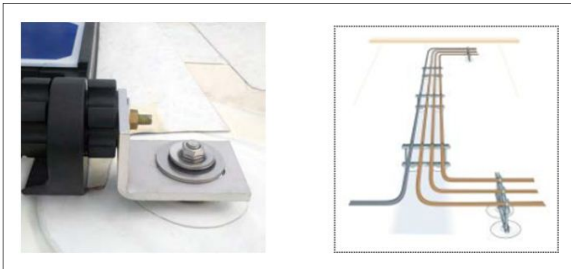
Fig. 2.1.1.9a and Fig. 2.1.1.9b. Examples of mechanical anchors used to secure equipment to the roof deck or roof framing
