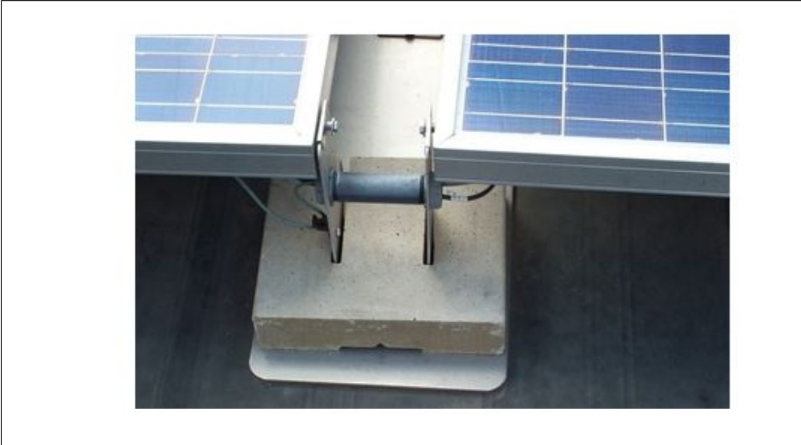
Fig. 2.1.1.11a. Slotted pedestal
