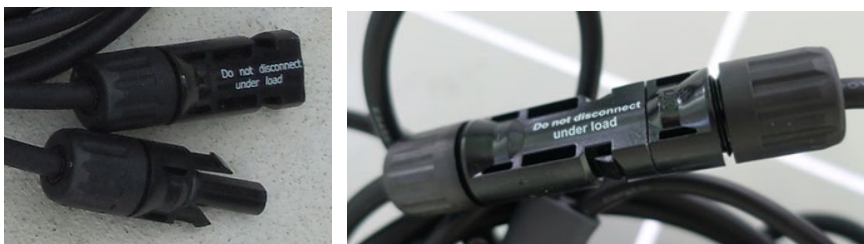
PV wire connectors - left photo disconnected and right photo connected. (Source: ZRS)
